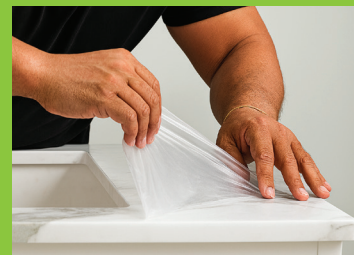
Fully polished benchtop surface with peel coat protection
